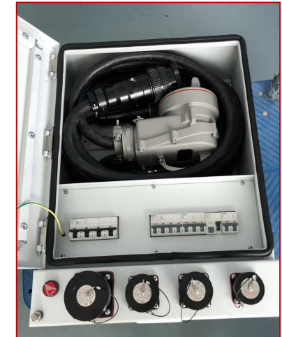
Integrated Shore Power Box
